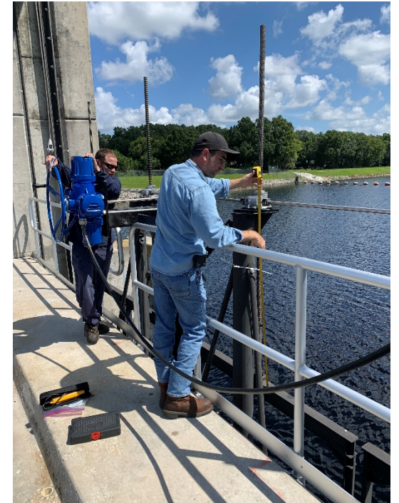
Setting the open/close limit switches
