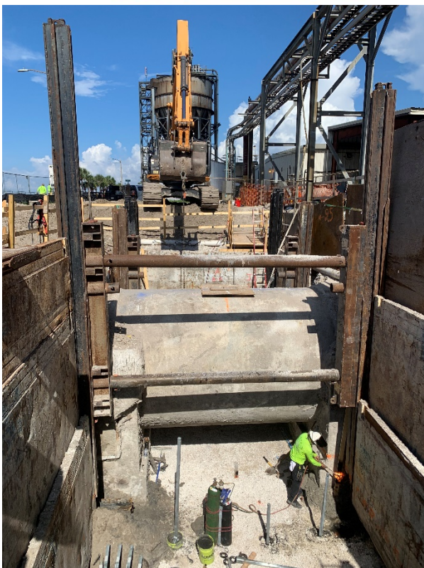
Excavate and expose the side of the tunnel
