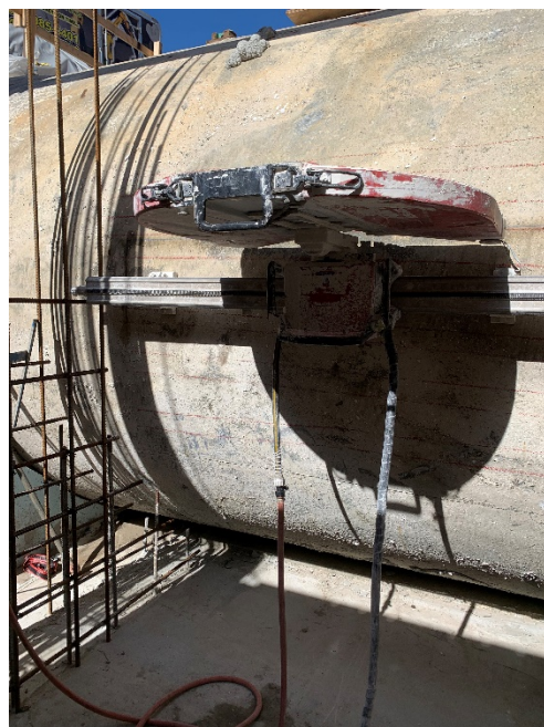
Cut 6' x 6' opening inside of tunnel
