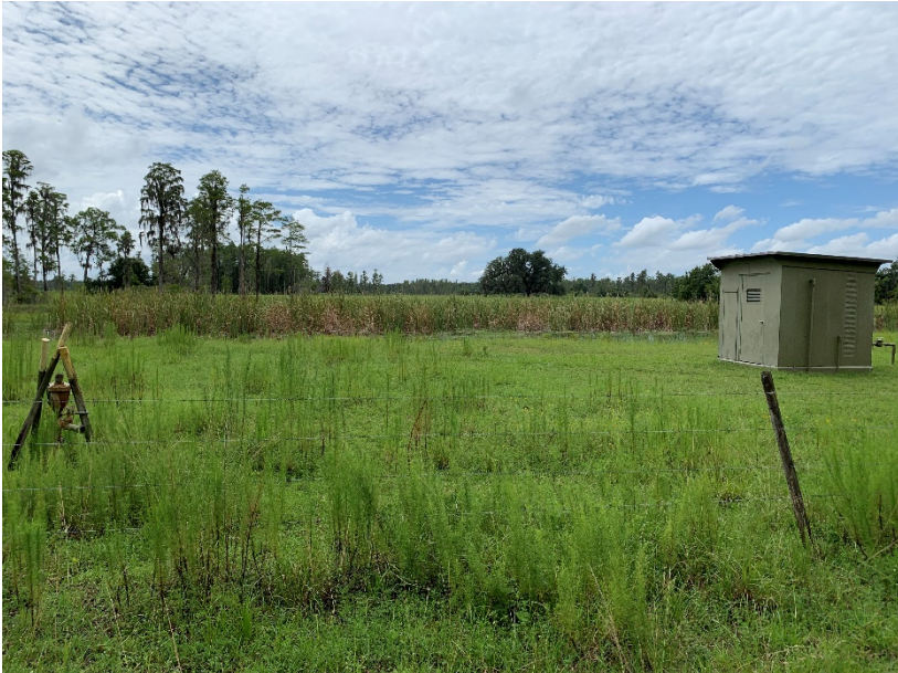
Wellhouse to be replaced
