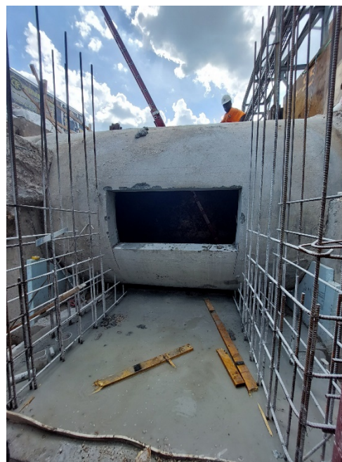
Cut 6' x 6' opening inside of tunnel
