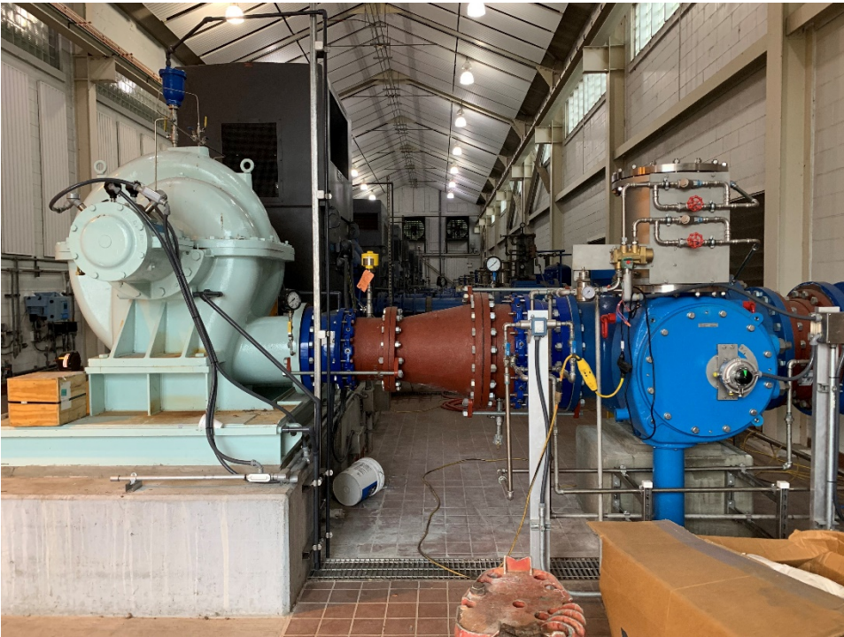
Pump and motor set in place
