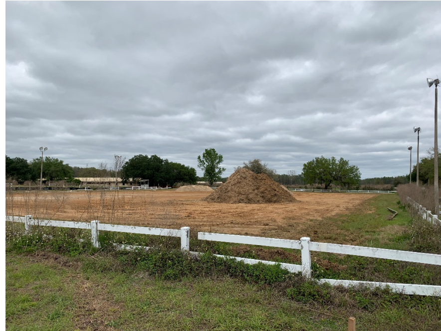
Clearing of Cypress Trails property
