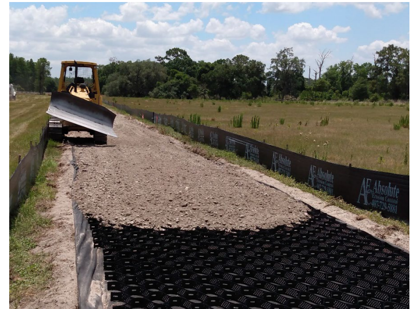
New access road installation
