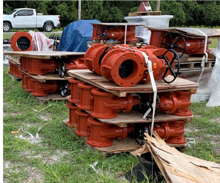
New gate valves to be installed
