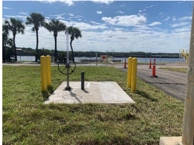
Desal Intake Phase 1
