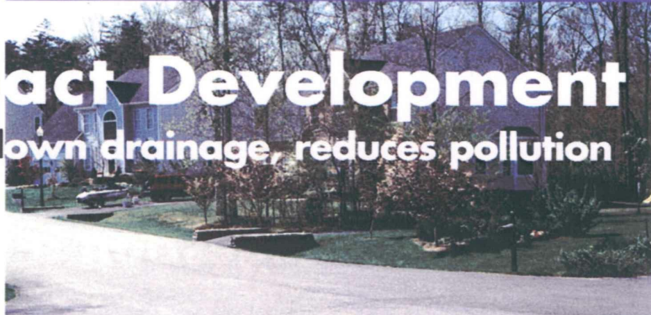
■ Low Impact Development seeks to maintain a region's hydrology even after development. In residential areas streets incorporate rain swales to help filter and slow runoff.
